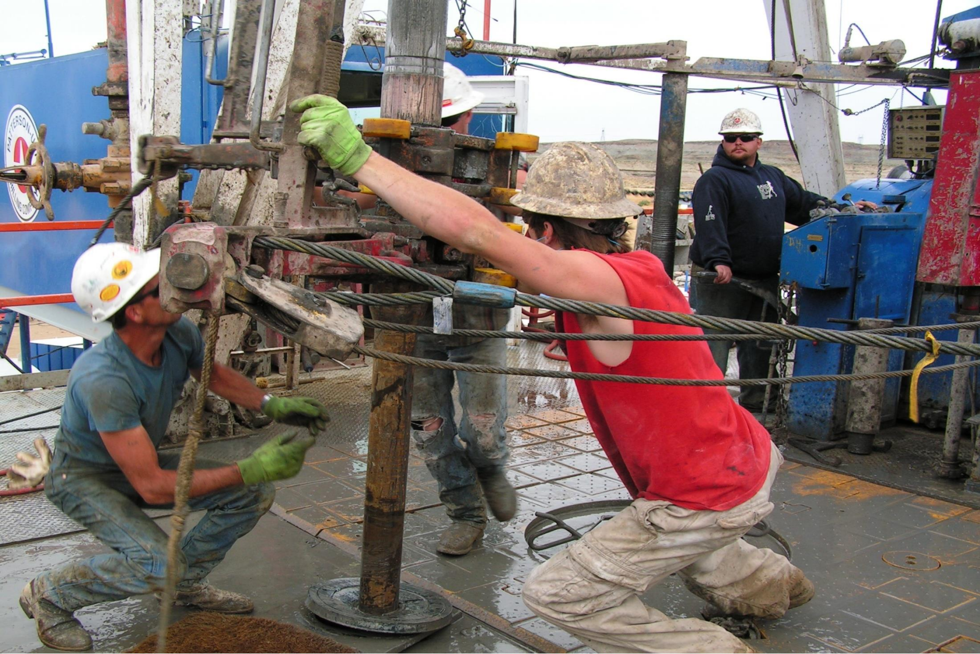
Derrick Platform - Vernal - Uintah County
